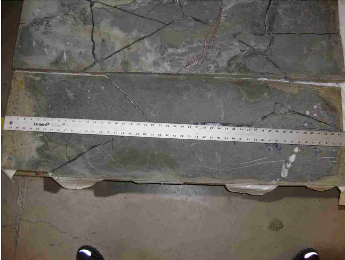
Figure 8.2.9: Failure patterns for short span 0% HSSFRC rectangular plates under longitudinal line load
