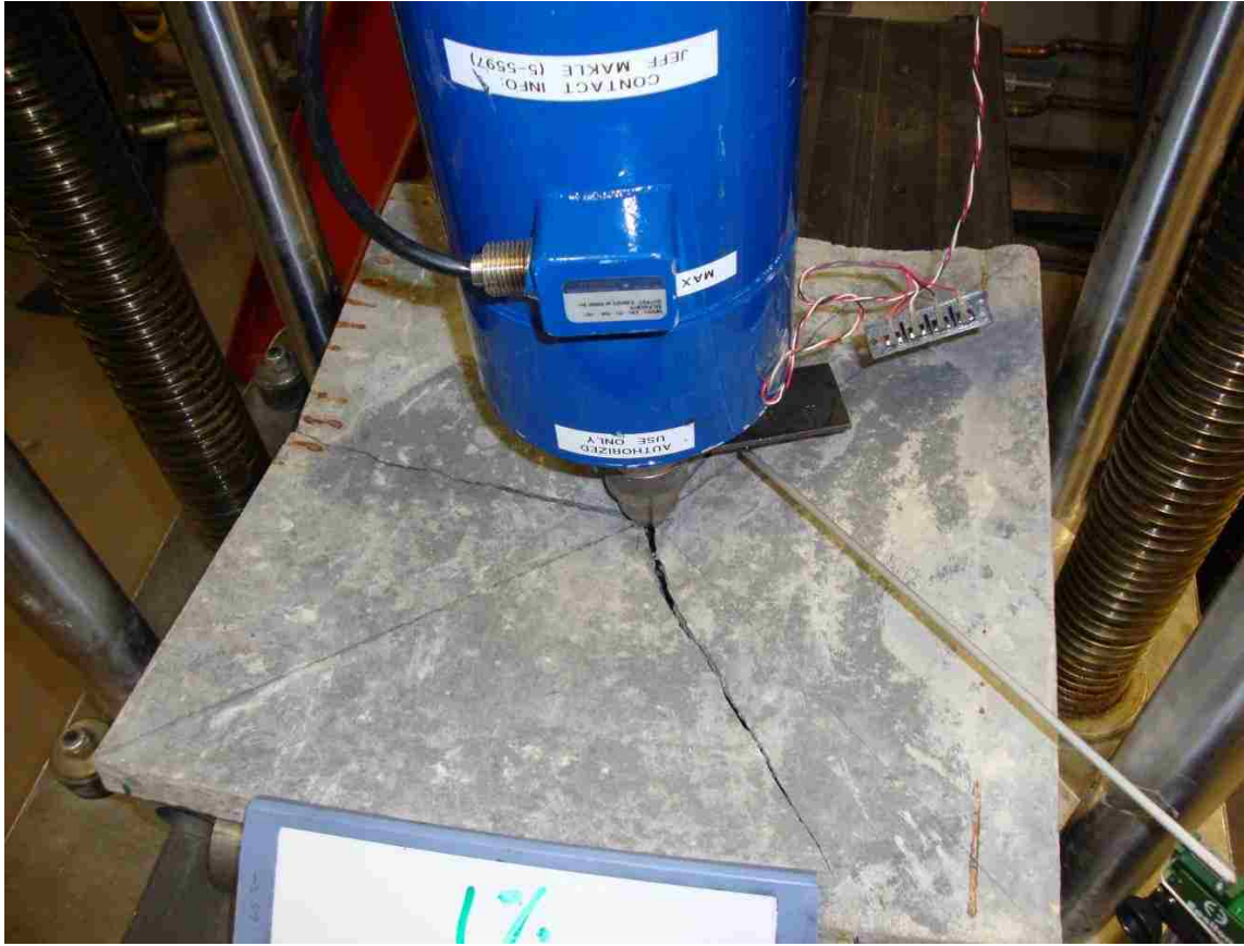
Figure 9.13: Crack patterns for 1% HSSFRC square plates under center point load
